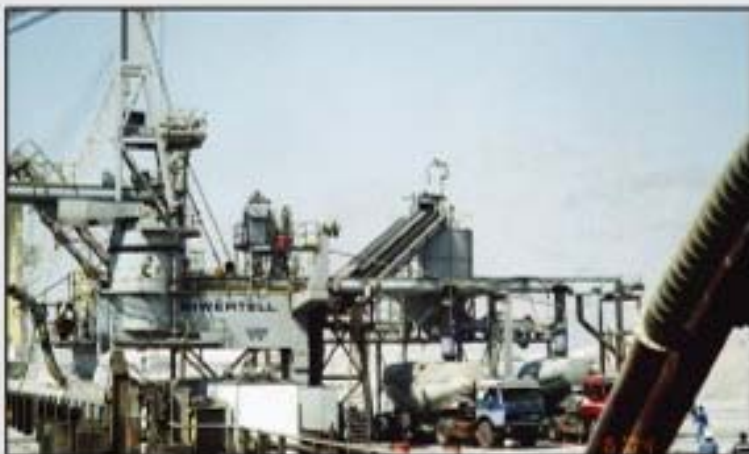
Bulk Cement Discharge
