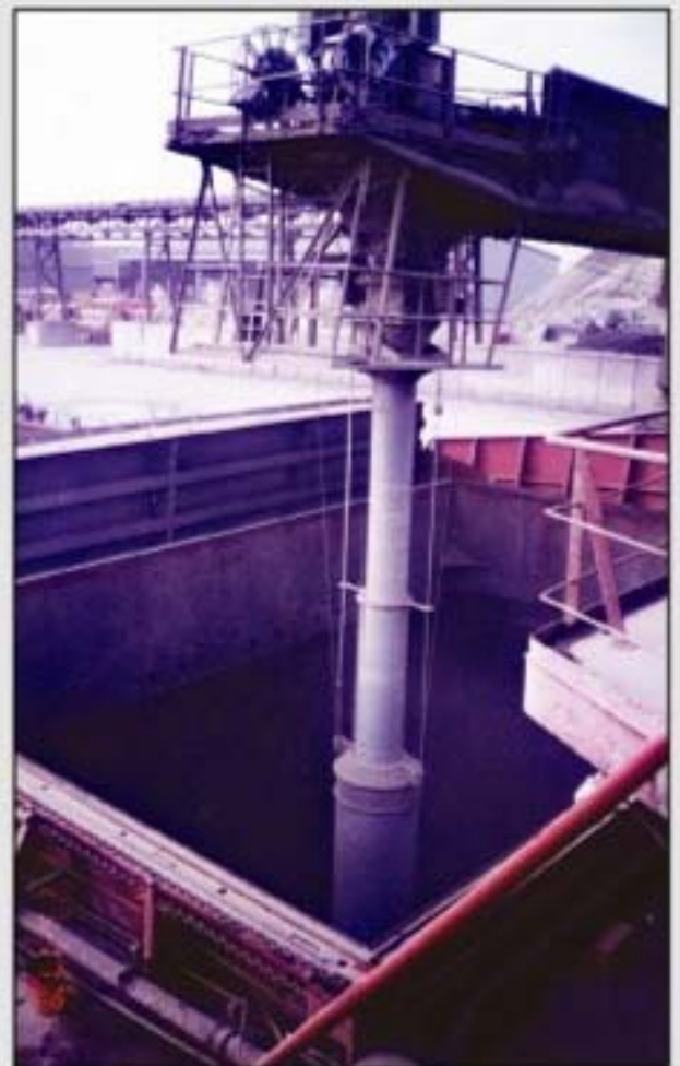
Bulk Cement Operations
